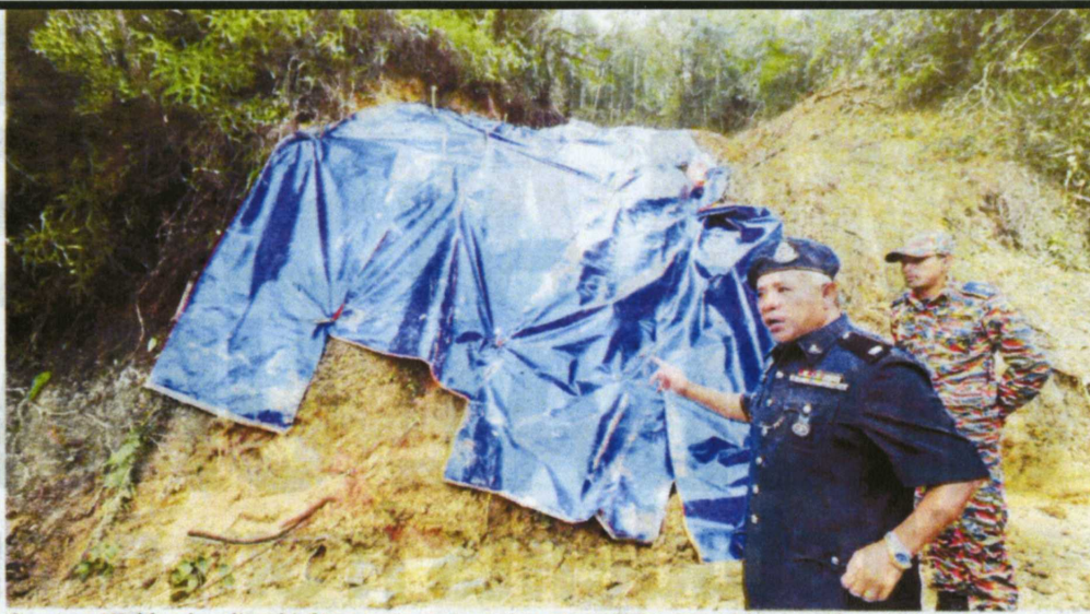
Cameron Highlands police chief Deputy Superintendent Hasadid A. Hamid (second from left) at the scene of the landslide near the Sharples Bungalow in Cameron Highlands yesterday. Pic by Muhaizan Yahya
